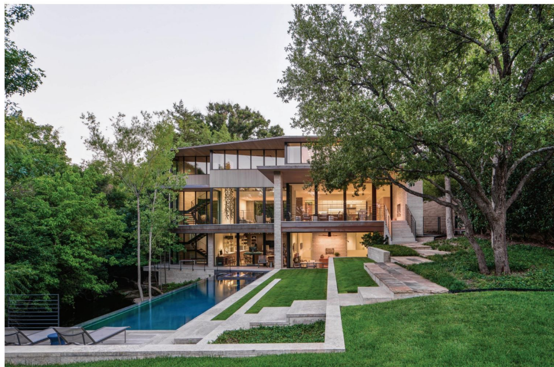
Embracing the natural surroundings, the home features bevel shell stone walls, siding and soffit in Douglas fir, and roofing and fascia in copper metal. The Richard Schultz 1966 chaise lounge in bronze is through Knoll with Kylix side tables through Janus et Cie. Landscape by Mesa Design Group, lighting by Byrdwaters Design, and custom builder Steven Hill all expertly realized the vision of this residence with Bodron/Fruit.
